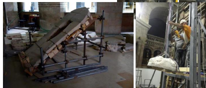
Removal of stone slab, transportation to conservation lab
