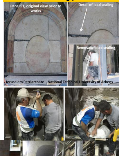
Dismantling process
